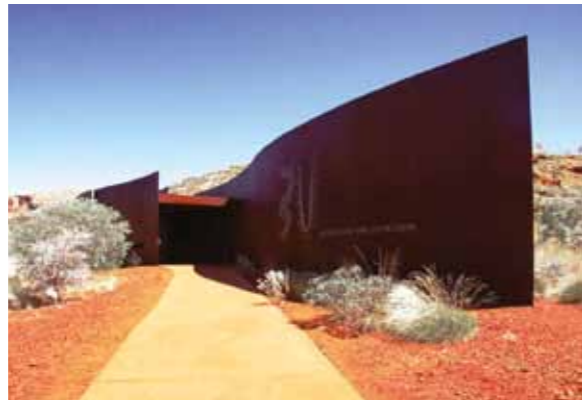
The Visitor Centre features free-standing, overlapping weathered steel wall panels derived from its context - an ancient landscape of rugged ranges and spectacular gorges
